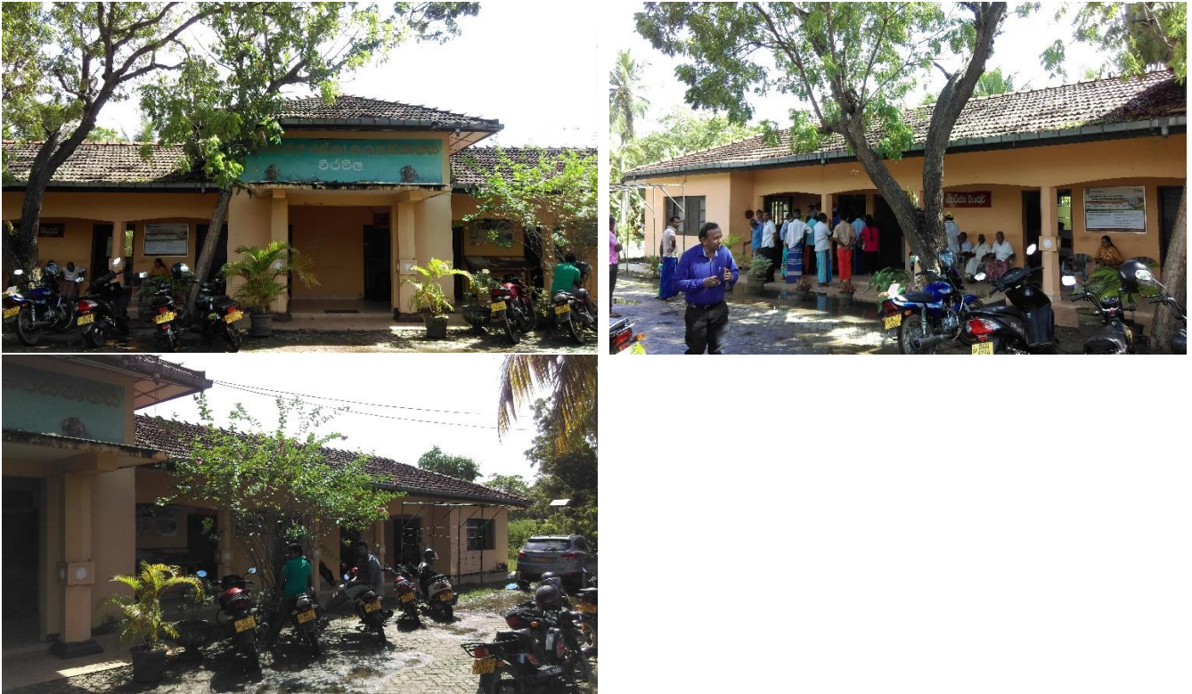
Old existing Agrarian Service Centre.
